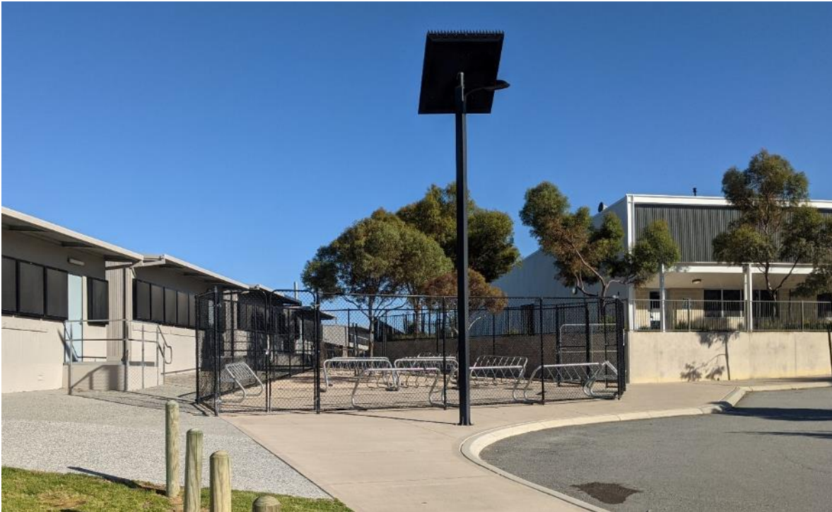
Figure 6-4 Existing Bike Bays
