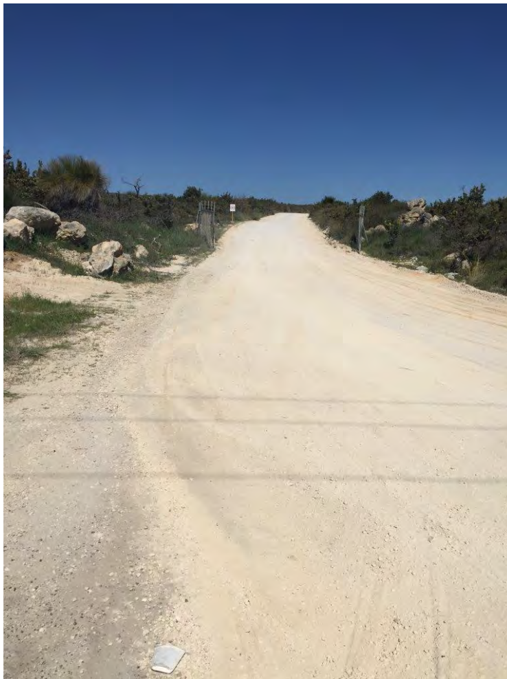
Access road from Wesco Road, on Lot 7
