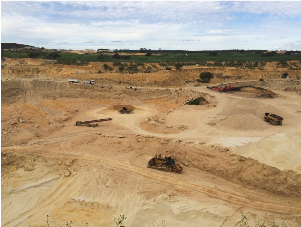
Plate 5: Site Operations within the Pit
