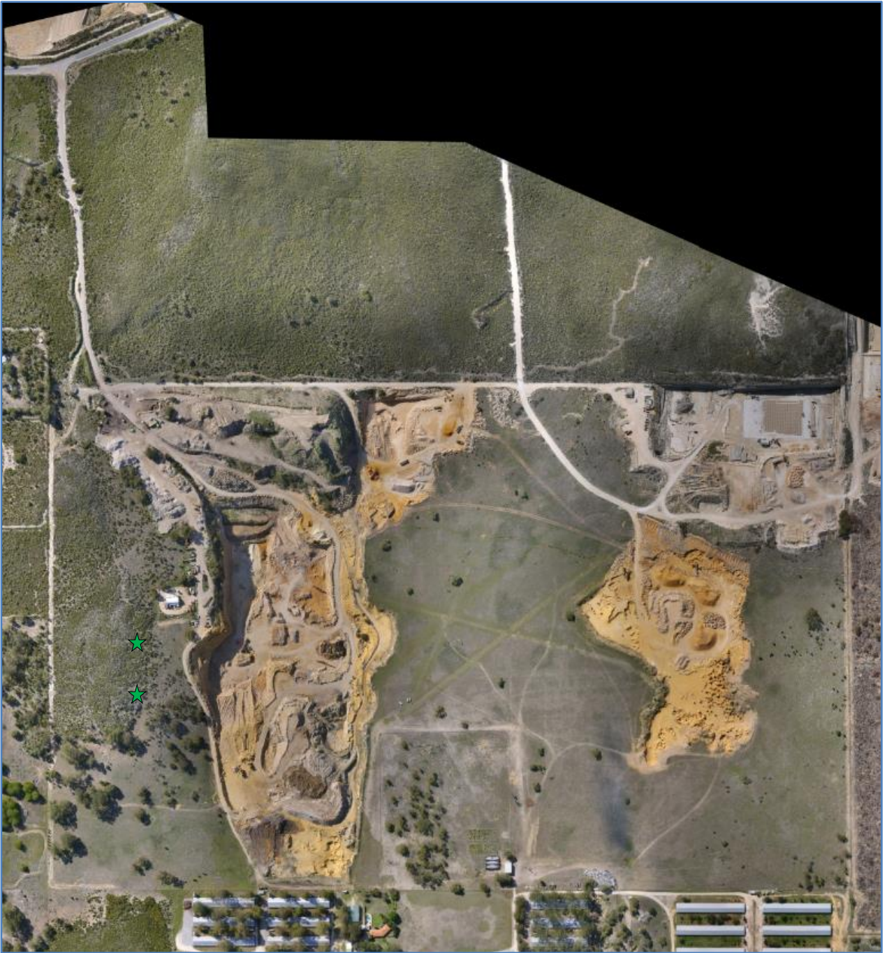
Figure 3. Very high resolution UAV derived orthophoto over the application area. The green stars represent the location of known karst structures (GSWA database).
