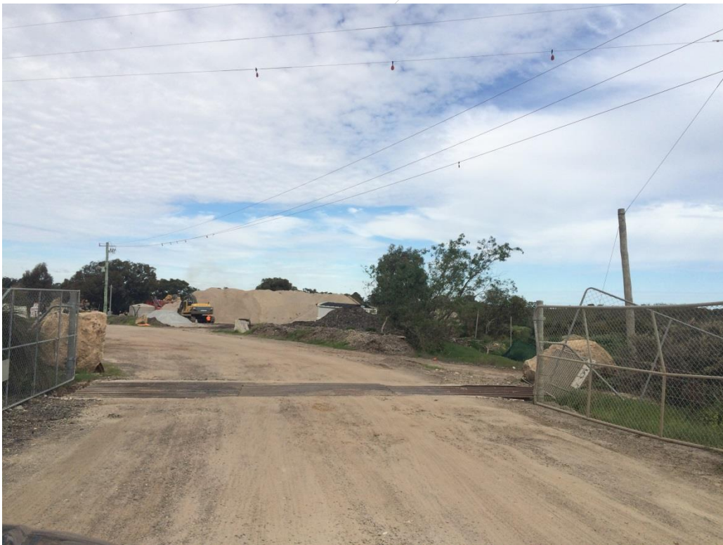
Plate 1: Lockable Entrance Gate
