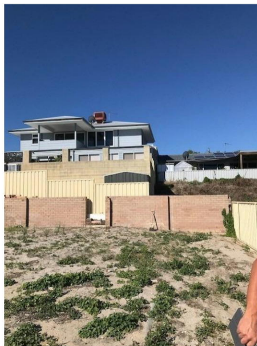
EXISTING REAR RETAINING, FENCING & REAR PROPERTY LEVELS
