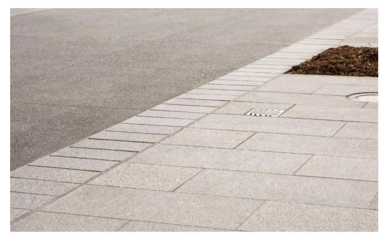
Road pavement flush with pedestrian footpath pavement with edge delineation
