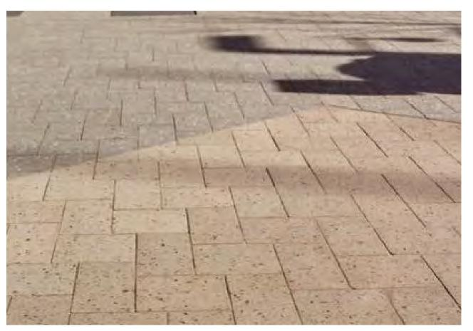
Tonal pavement variation between road pavement and pedestrian footpath pavement using small paving size and pattern
