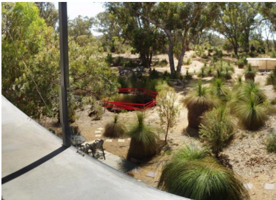
Figure 4a – Breakwater Drive, Two Rocks. View of sinkhole from balcony of residence
