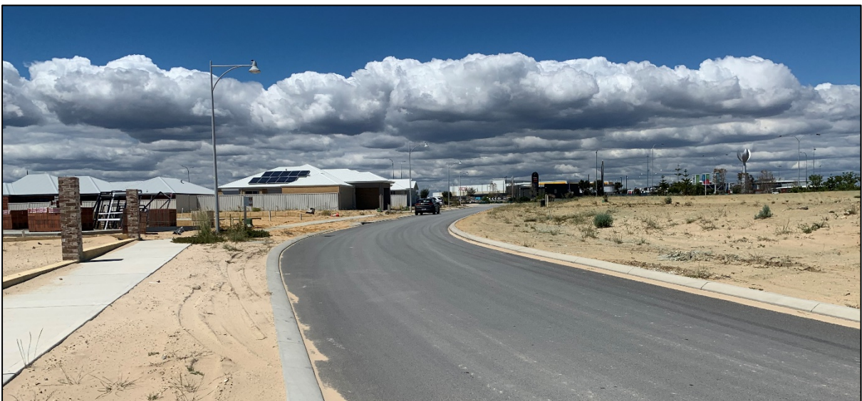
Photograph 8: The adjacent properties north of the development site, as viewed from the west.
