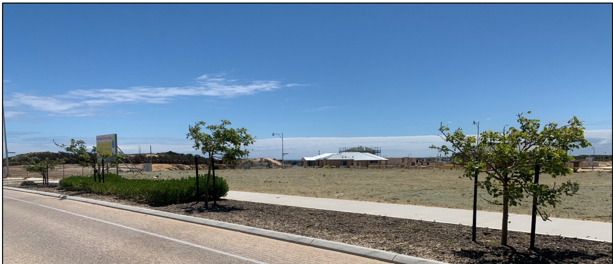
Photograph 1: The southern frontage of the development site, as viewed from the south (on Hawksbill Drive).
