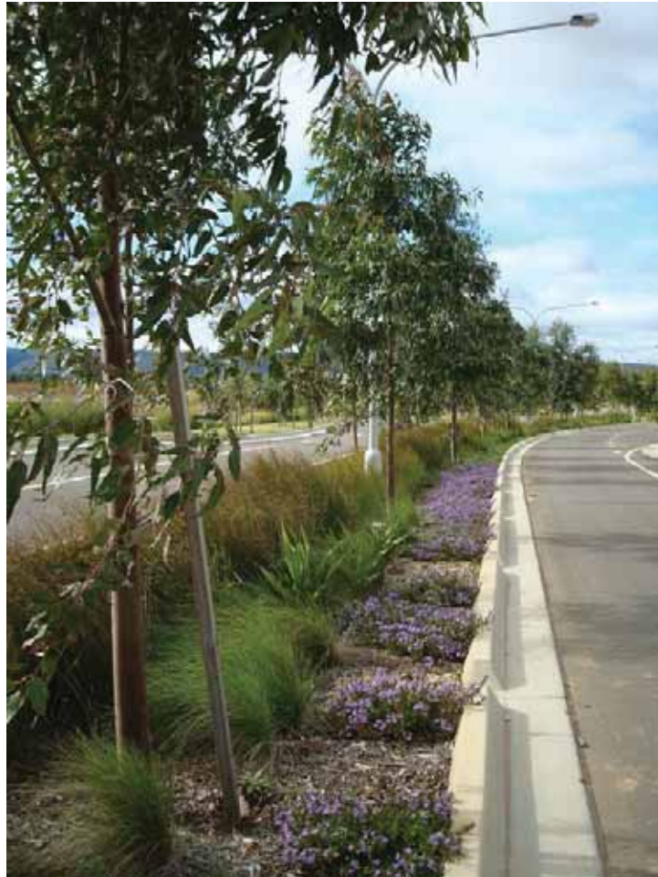
Plate 3: Indicative median swale design
