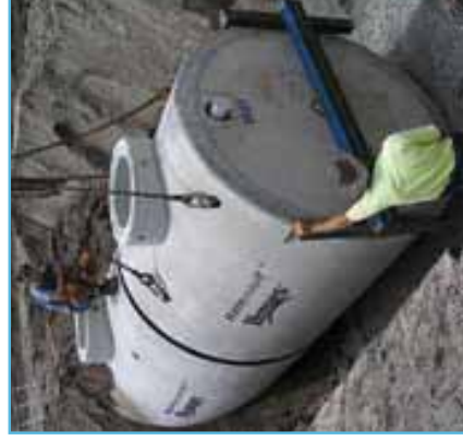
Concrete underground tank
