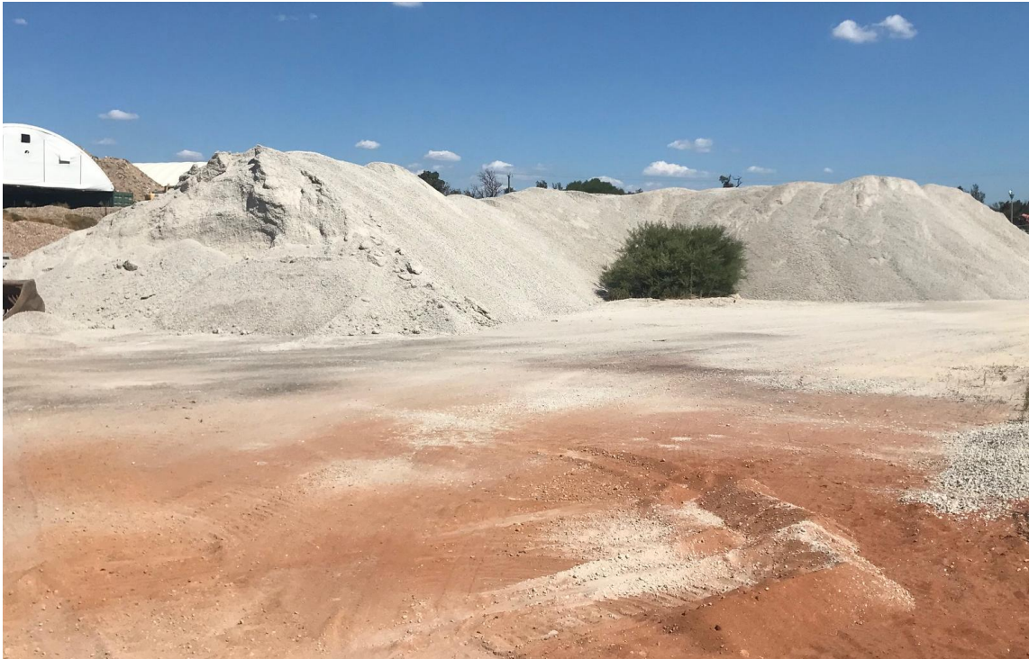
Figure 3-5 Stockpile Acting As a Noise Bund
