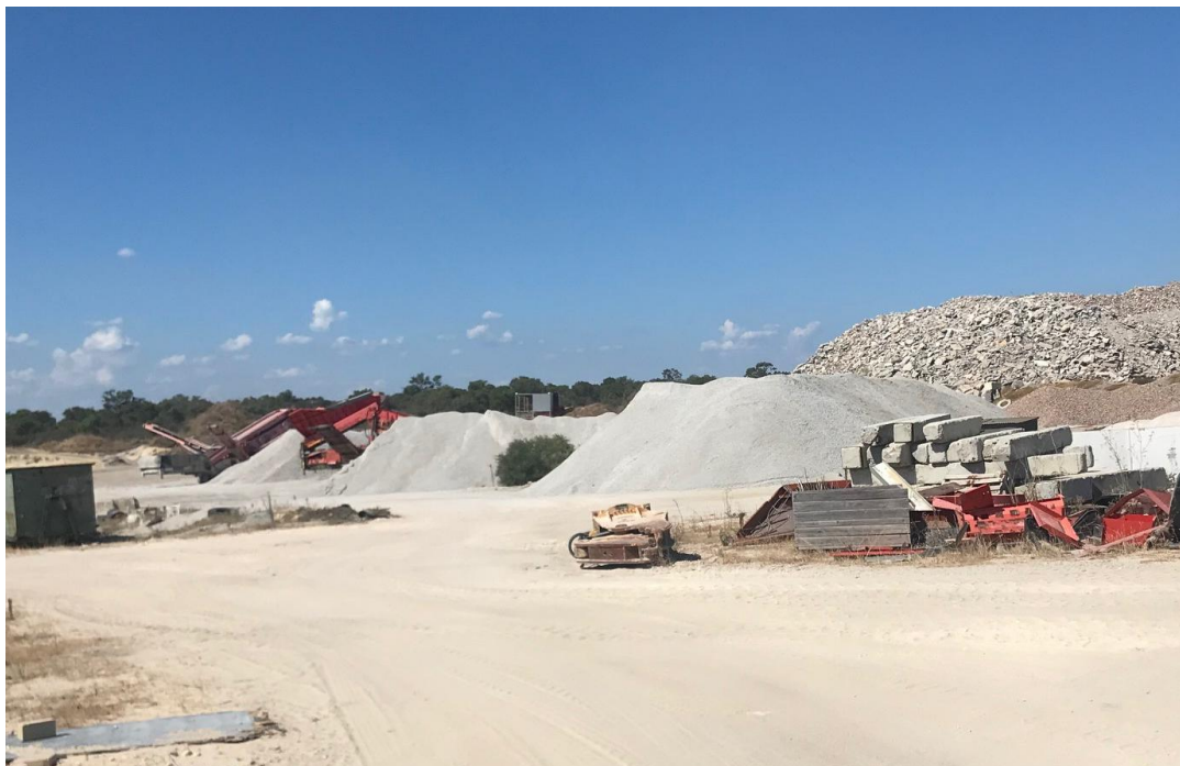
Figure 3-4 Plant With Surrounding Stock Pile Noise Bunds
