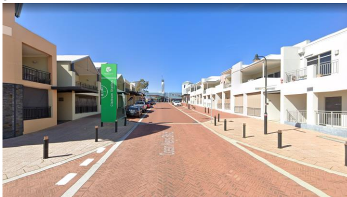
Figure 15 – Looking East on Ocean Keys Boulevard towards the train station
