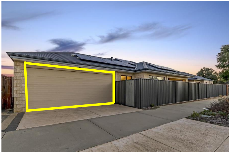
Indicated in the above picture, showing you the double garage entrance to the parking at the property.
