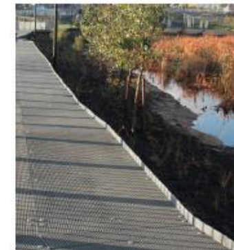
UV stabilised Fibre Reinforced Plastic (FRP) grating and kick-rails to be used for the bird hide boardwalk
