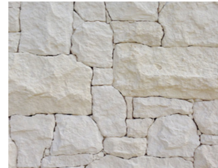
Limestone rubble cladding
