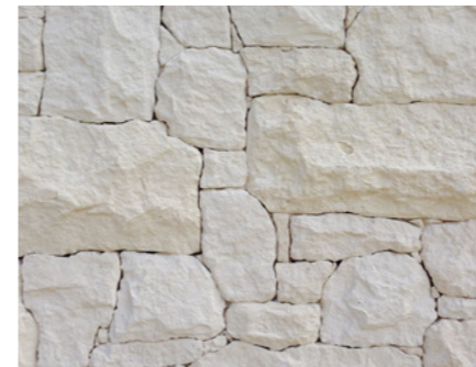
Limestone rubble cladding
