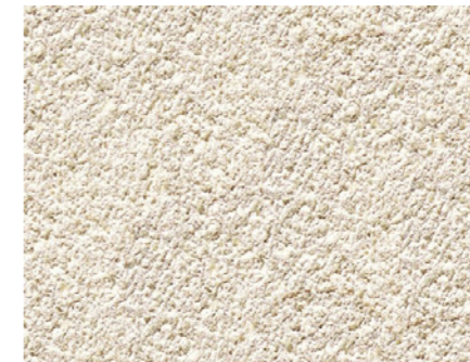
Rendered masonry walls
