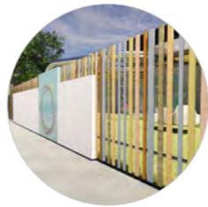
Masonry & Pre-finished Aluminium Fence
