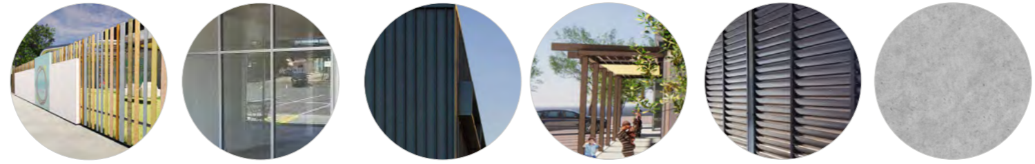
Masonry & Pre-finished Aluminium Fence Aluminium Framed Glazing Pre-finished Metal Cladding Pergola Structure Pre-finished Aluminium Louvres Painted Cementitious finish
