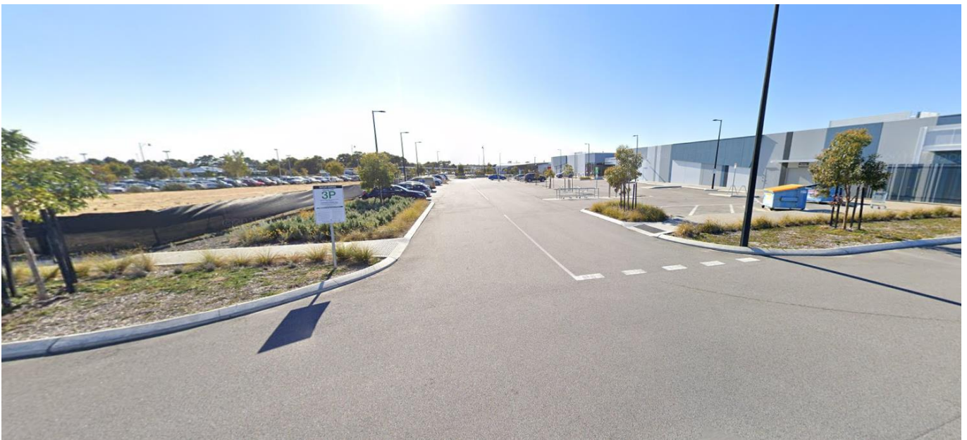
Figure 8 Existing access from the Existing Connector Road into the Butler Central Shopping Mall northern car park – the Butler Childcare Centre is proposed to occupy the vacant Lot on the left side of the Streetview image (source: Google Streetview)
