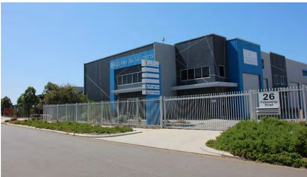
Figure 6-17 Two storey articulated building façade which appropriately address the street and public realm
