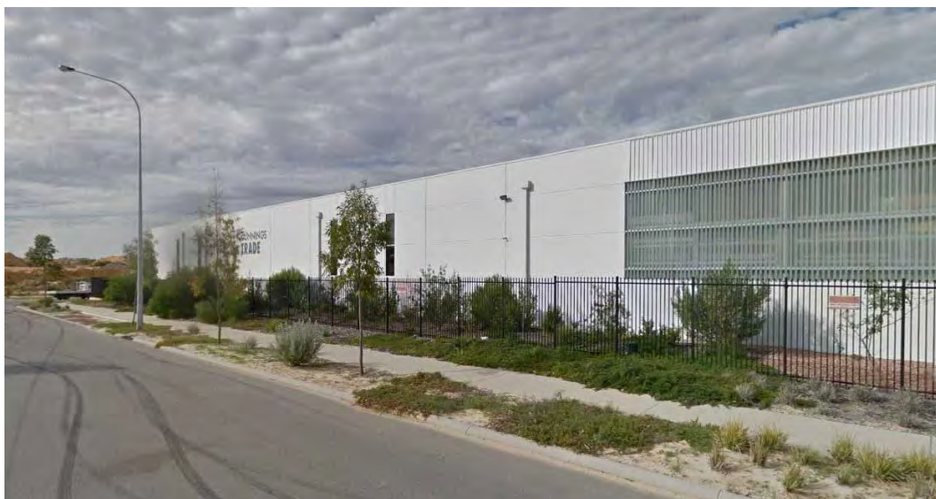
Figure 6-6 Example of building close to street screening service yard behind
