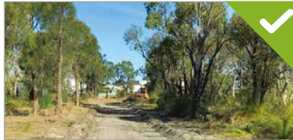
A compliant firebreak needs to be 3m wide and trafficable with a vertical clearance of not less than 4m.
