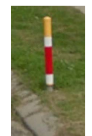
DETAIL 2 - FRANGIBLE BOLLARD BEHIND MOUNTABLE KERB
