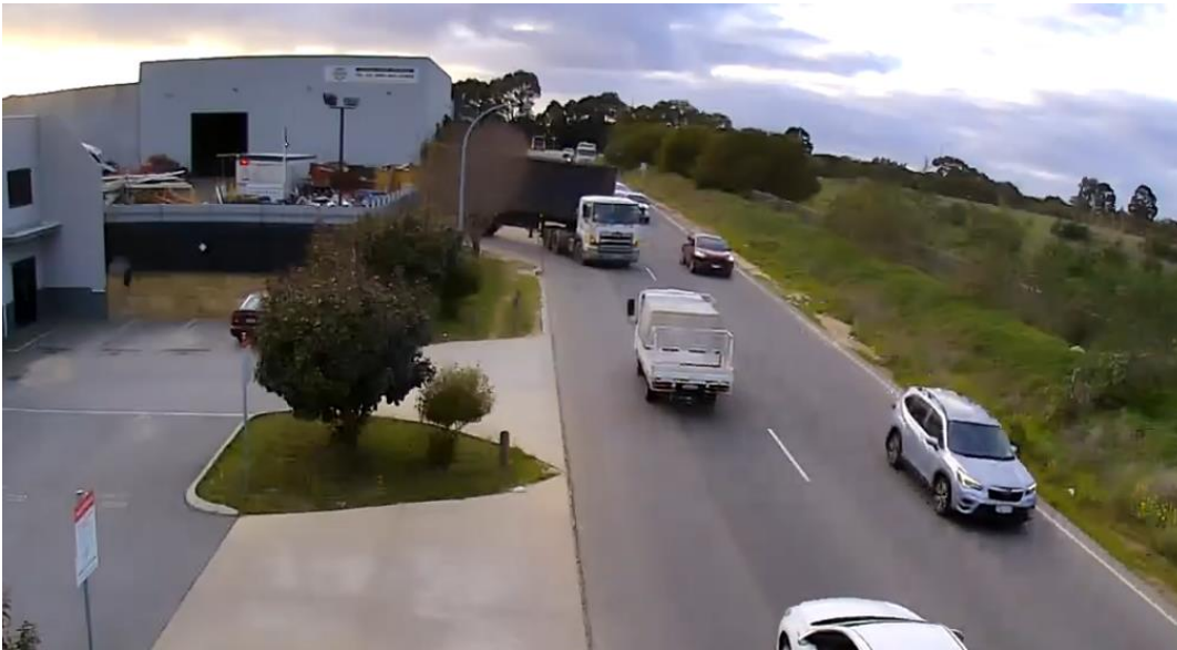
Figure 7.2 – Truck Reversing into the Demolition Site
