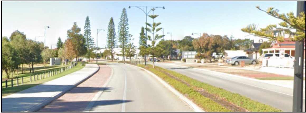
Figure 5: Eastbound view of Kingsbridge Boulevard
