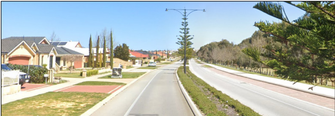
Figure 4: Westbound view of Kingsbridge Boulevard
