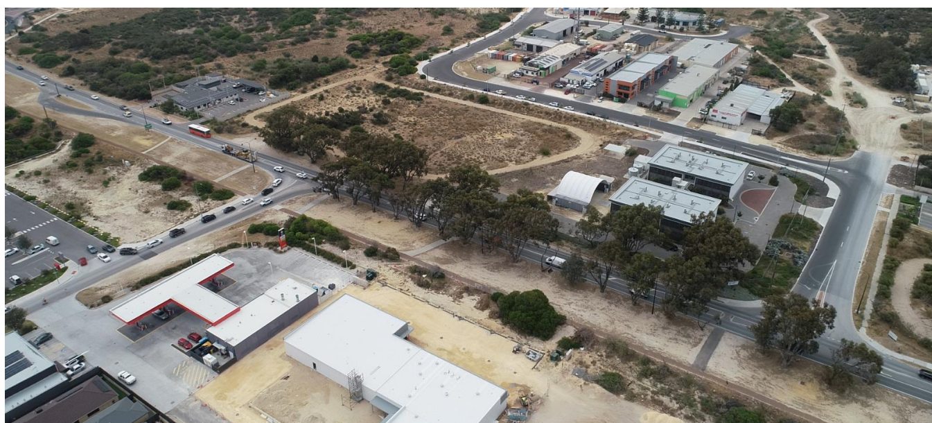
Figure 10: Existing traffic queue on Kakadu Rd (Monday 6/11/23 at 3:00pm)
