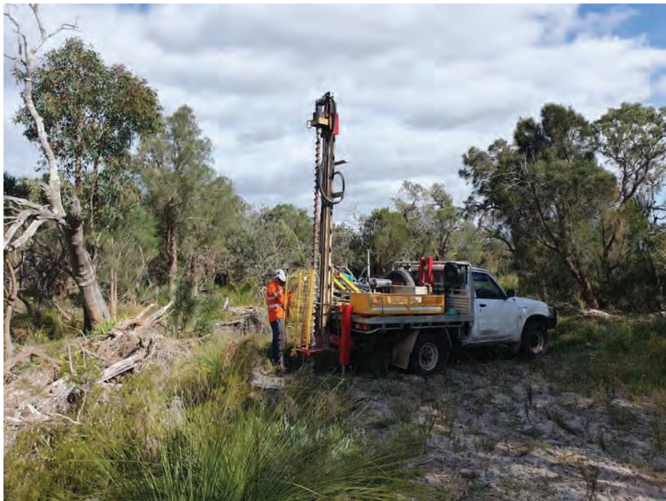
Photograph 5: Drilling borehole near IT07
