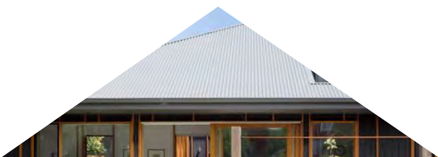
Light grey corrugated metal roof
