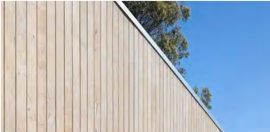
Timber-look cladding on stud system
