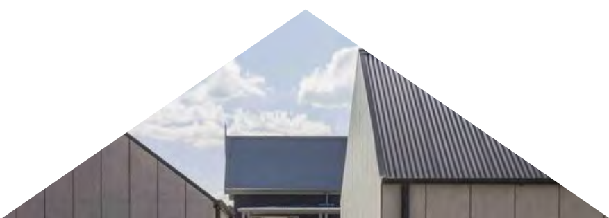
Light grey corrugated metal roof
