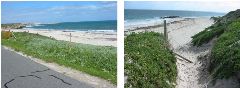
Poor and damaged fencing in study area
