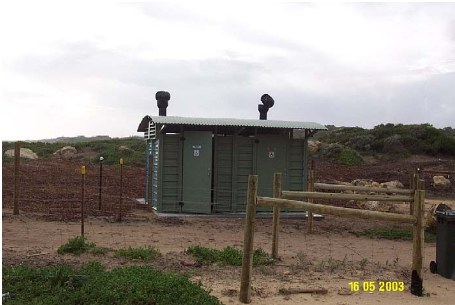
Composting Toilet at Two Rocks
