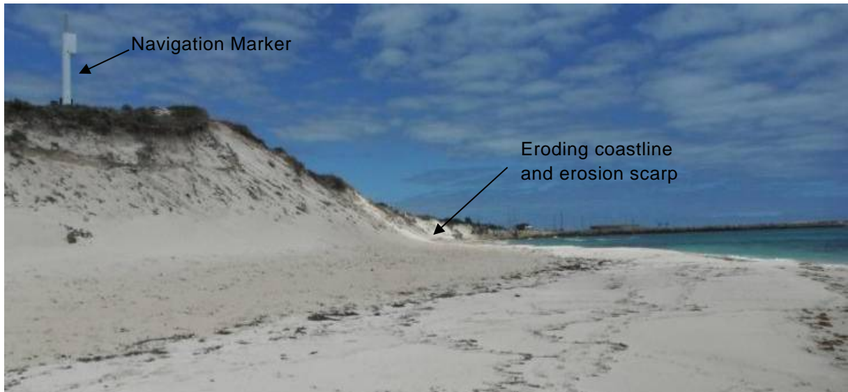
Figure 2.6 - Erosion North of the Marina (6/12/12)
