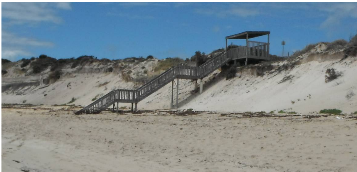
Figure 2.7 - Erosion Near the Sceptre Court Stairs & Viewing Platform (6/12/12)
