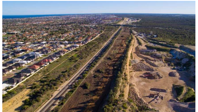
Aerial view of the future freeway alignment looking north towards Hester Avenue.
