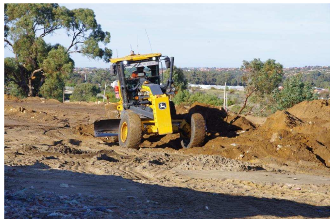
Water cart and grader in operation at the worksite.
