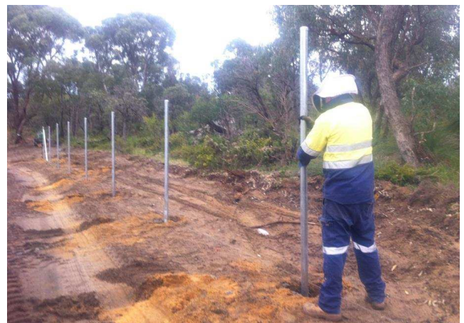
Installation of permanent fauna fencing.
