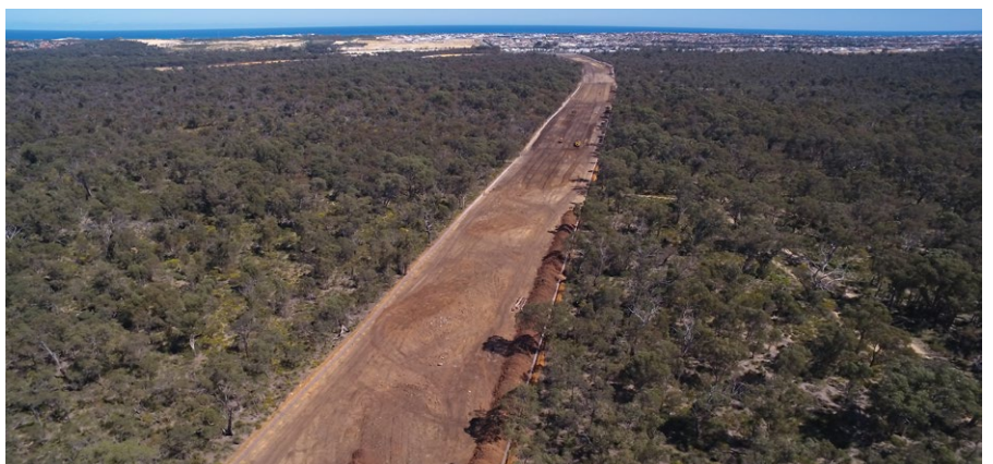
Aerial view of Neerabup Road Extension looking west towards Clarkson. Earthworks are underway to build up the levels along this new section of road.
