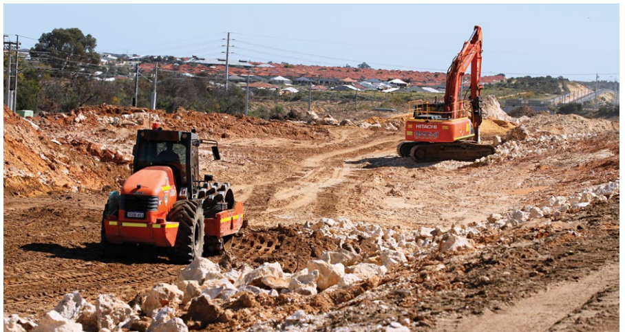
Earthworks, involving trucks, scrapers, excavators and rollers, are underway across the entire project area to establish the levels of the freeway.
