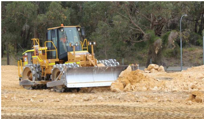
825 Compactor in operation near Tamala Park, spreading and compacting material.
