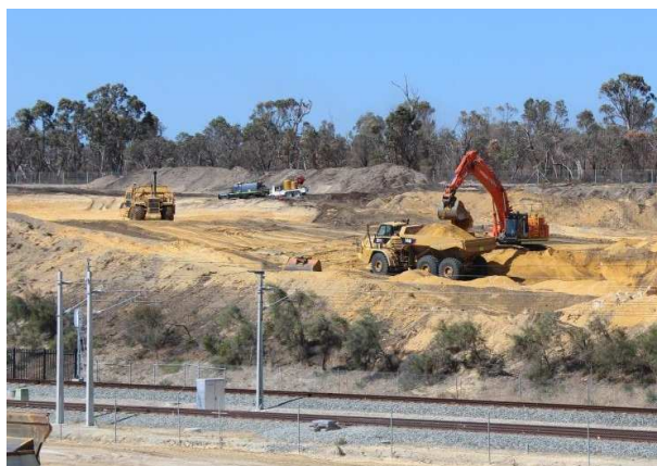
Earthworks continue near Clarkson Train Station.
