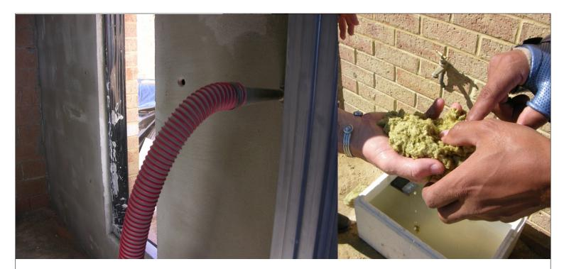
Cavity insulation is a proven way to keep your home warmer in winter and cooler in summer. Given that up to 25 % of heat gain and loss in a typical brick home in Perth can be through the walls, it makes sense to prevent this waste of energy through incorporating cavity insulation.
