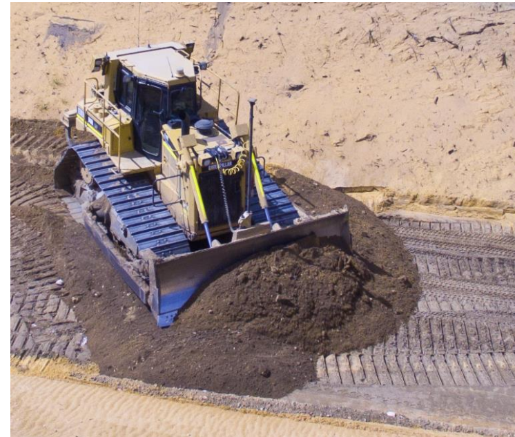
Earthworks at Neerabup Road.
