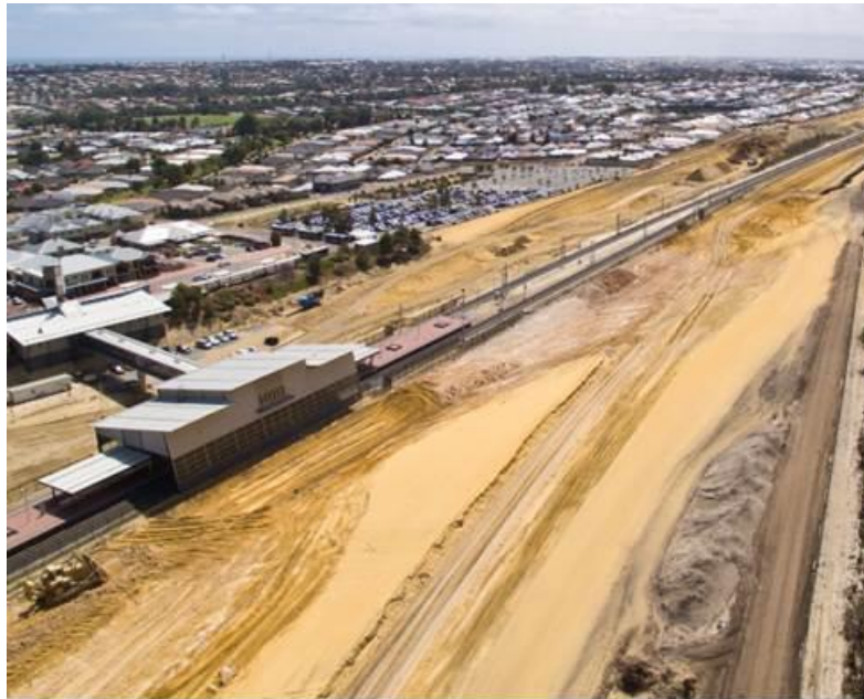
Progress of works near Clarkson Station.
