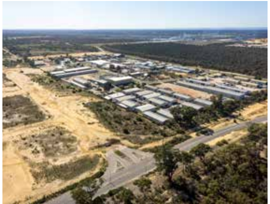
Aerial view of existing Neerabup Industrial Area
