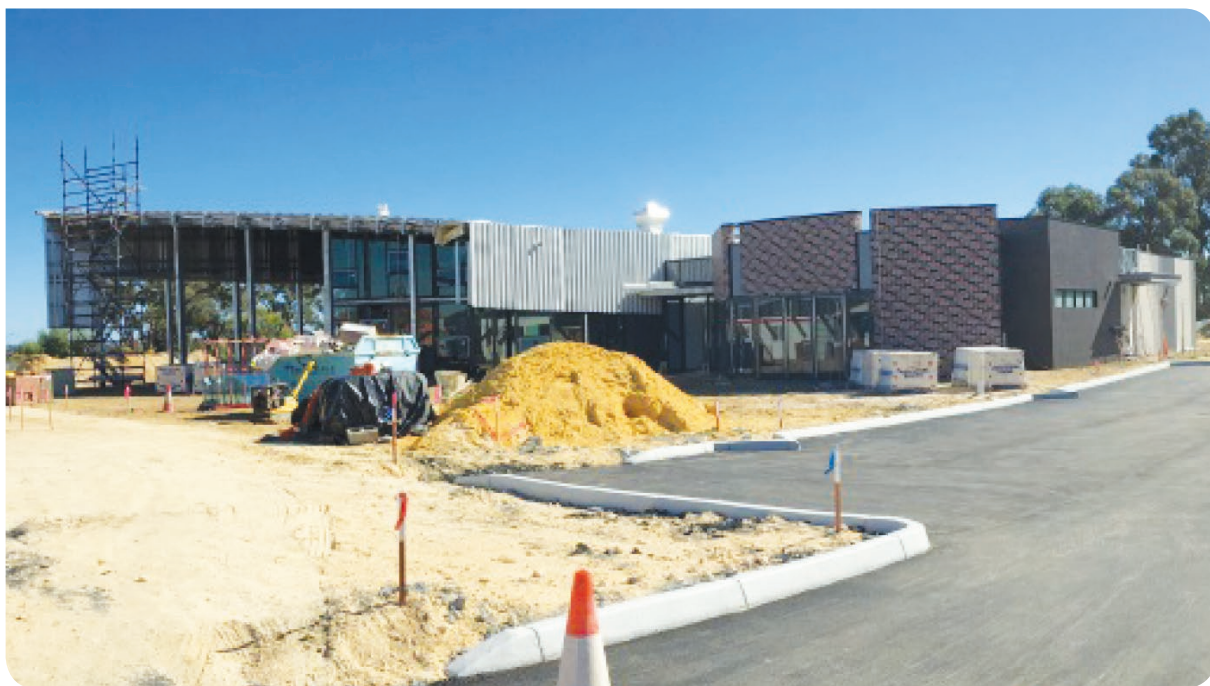
The Pearsall Hocking Community Centre under construction.
