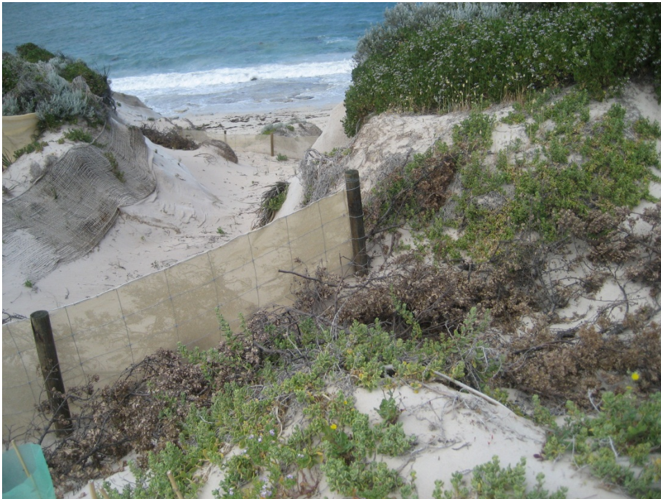
Plate 11 Examples of coastal stabilisation techniques, including brushing, sand trap fencing and jute matting.
