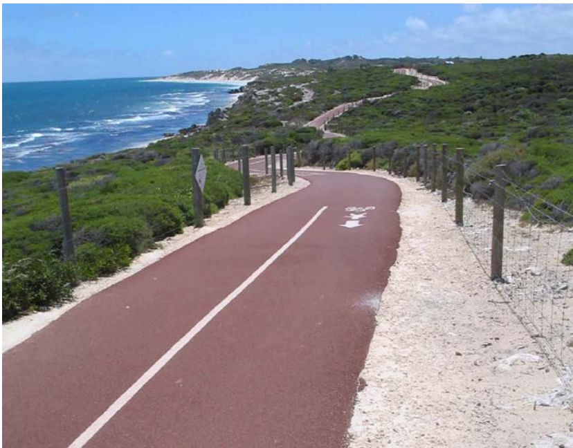
Plate 16 Example of a universal pathway system with shallow gradients over existing landform
