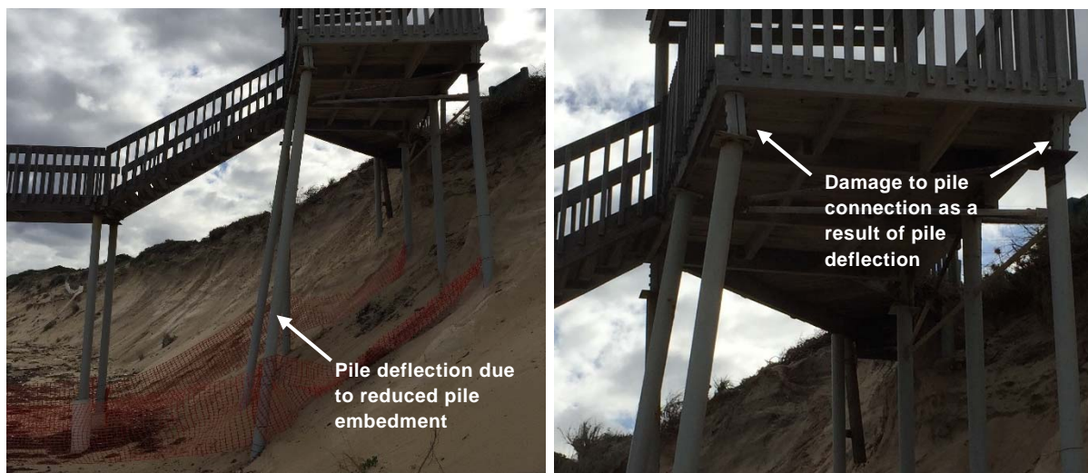
Figure 2.2 Pile Deflection & Damage to Pile Connections
