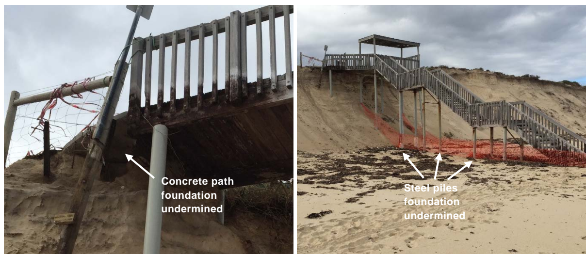
Figure 2.1 Undermined Concrete Footpath & Pile Foundations
