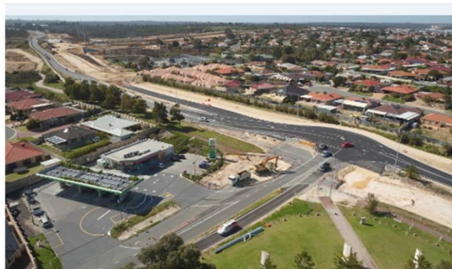
Above: Progress of construction of the new Hester Avenue/Ridgewood Boulevard roundabout
