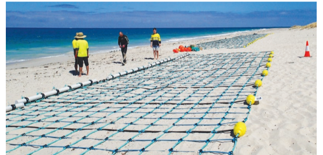
Undertaking the installation of the 300m eco-friendly barrier at Quinns Beach.
