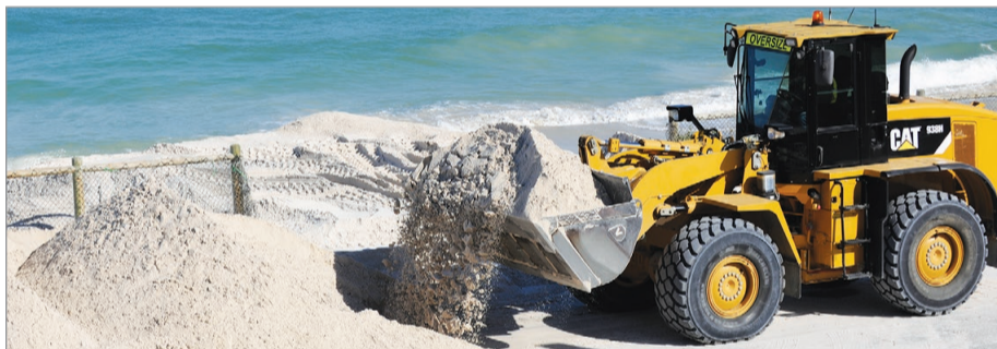
Coastal protection works are a feature of the 2017/18 capital works program.
