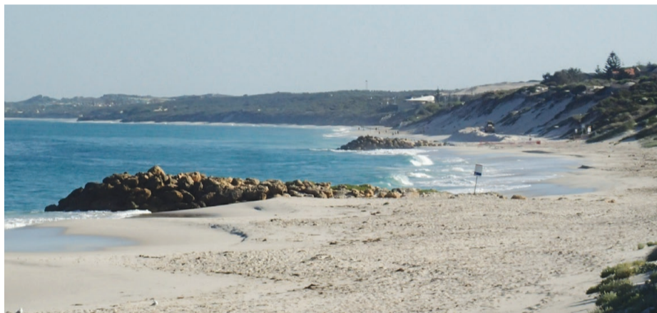
Groynes are due to be extended and another added at Queenscliff Park.
