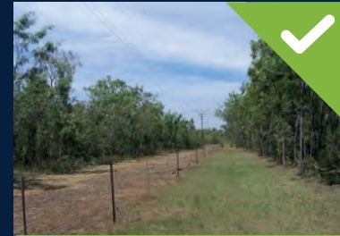
Compliant: grass slashed to ground level
