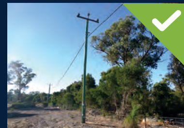
Compliant: cleared buffer zone around power poles
