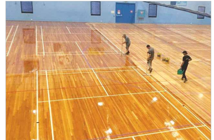
Recoating the courts at Kingsway Indoor Stadium.
