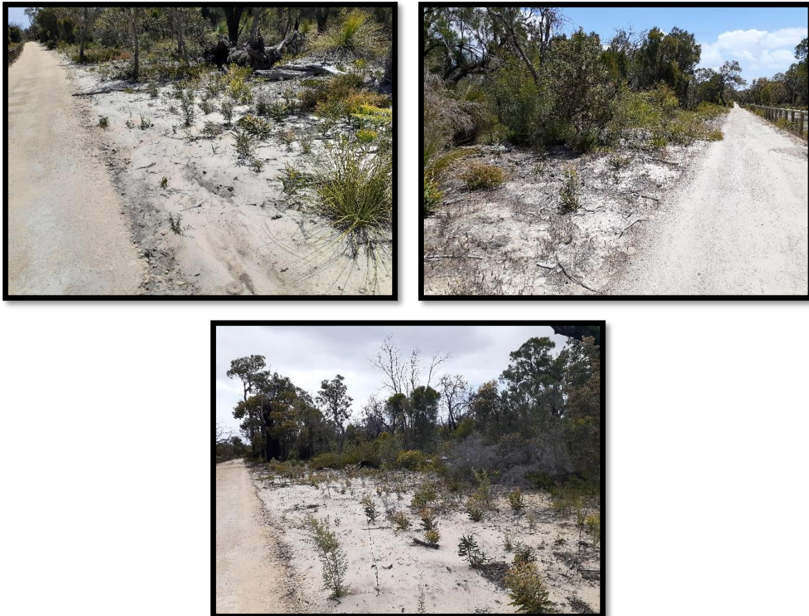
Plate 6, 7 and 8: Dieback Inspection
