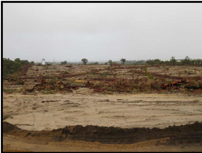
Plate 1: Clearing of Stage 1
