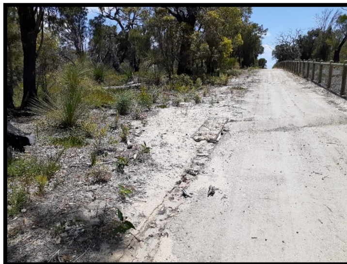
Plate 5: Crushed limestone Firebreak with installed Caged Gabions
