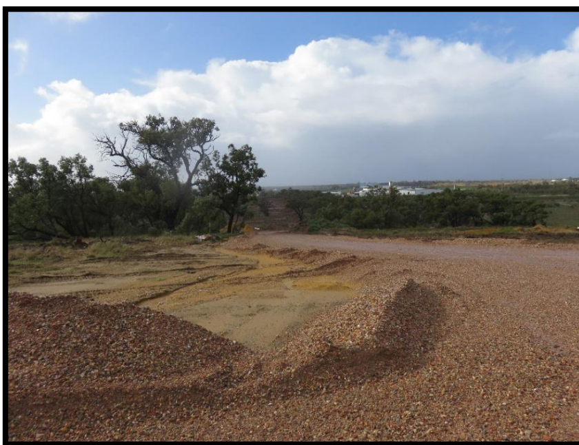
Plate 2: Crushed Brick Access Road
