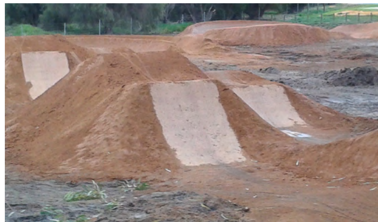
DETAIL A CONCRETE JUMP LIP- TYPICAL DETAIL
