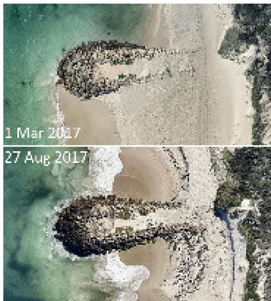
Figure 5.15 – A groyne at Quinns Beach, shown at the end of summer (top) and during winter (bottom) (Cardno, 2018).
