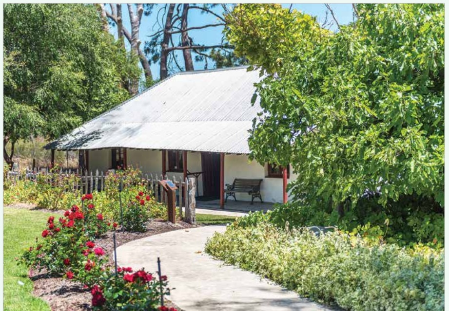
Completed in 1860, Cockman House in Woodvale was a family home for three generations.
