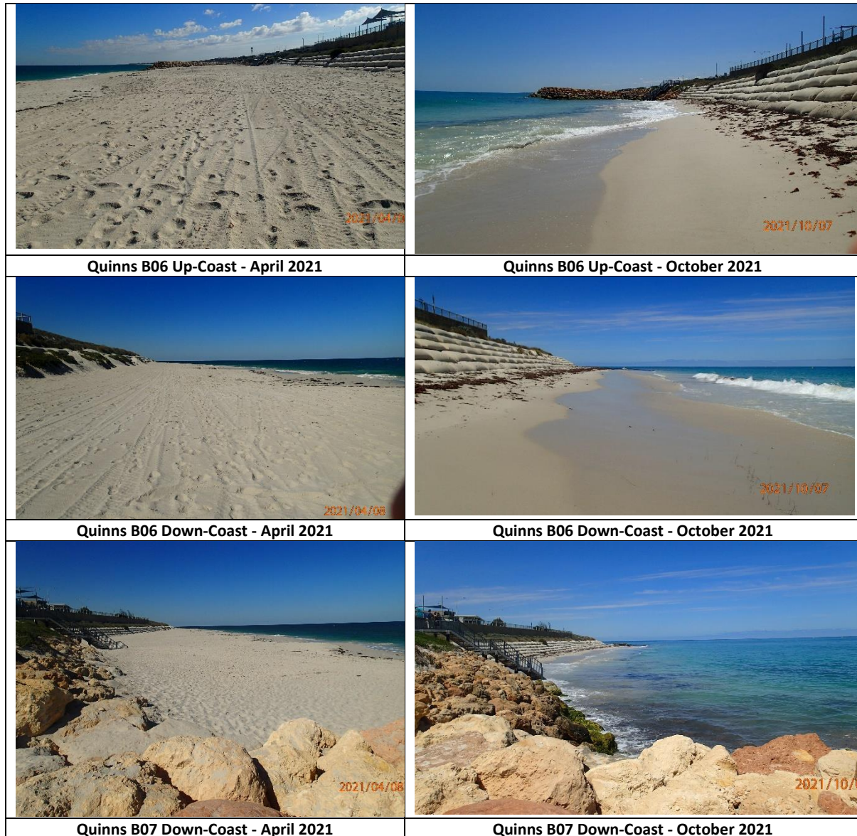
Figure 4-9 Major erosion over winter 2021 at Quinns B06 Up-Coast, Down-Coast and Quinns B07 Down-Coast.
