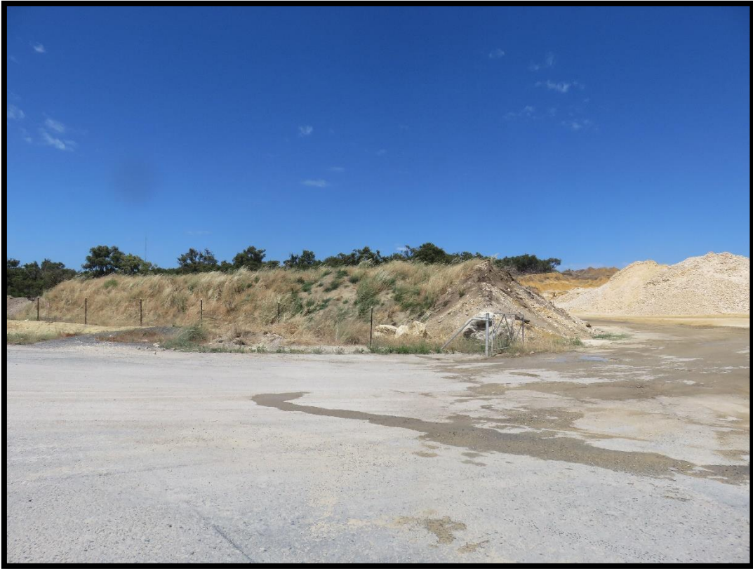
Photo 7: Weeds on stockpile
