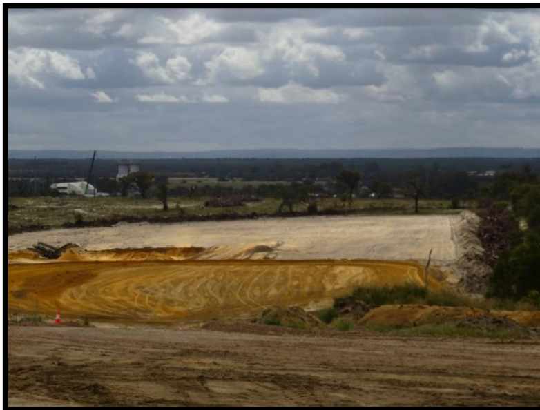
Plate 5: Extraction and Contouring Operations Stage 2 October 2021
