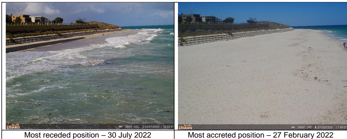
Figure 6-3 Most receded and most accreted shoreline position to the south of Quinns Groyne 1 during the study period.
