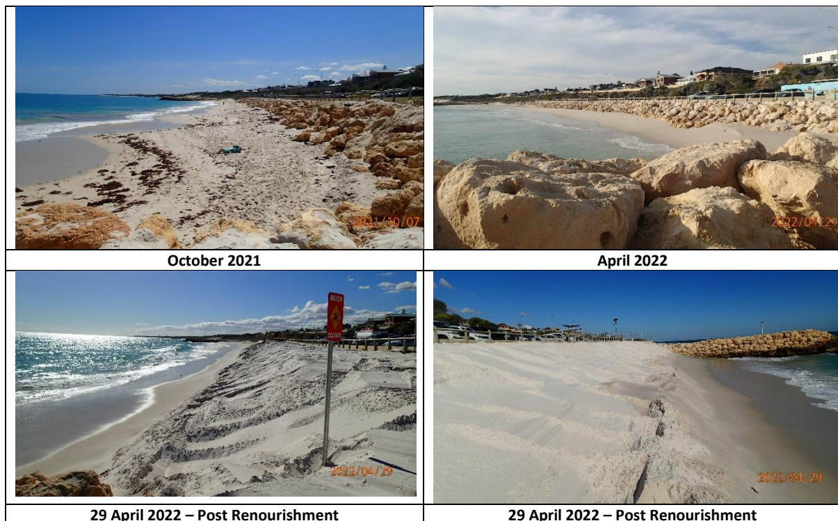
Figure 4-6 Major erosion over summer 2021/22 at Quinns B07 Up-Coast.
