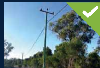
Compliant: cleared buffer zone around power poles
